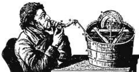
FIG. 2. Method of breathing oxygen and absorbing carbon dioxide used by Ingen Housz in 1783. "Several hours before using the dephlogisticated air one shakes in the water of the bucket a good piece of quicklime." Lacking exact knowledge of Fontana's method of proceeding, . . . "I devised a method which succeeded for me just as well." Nouvelle Recherches , 1785. (Illustration taken from Ingen Housz' original work.)
