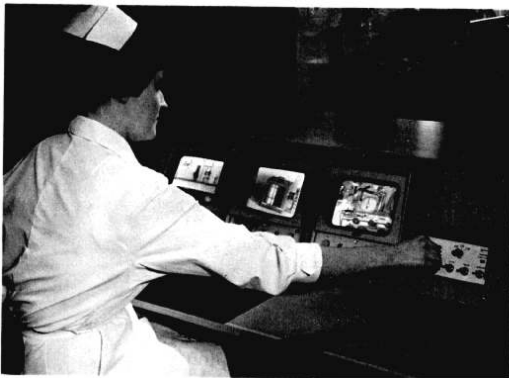
FIG. 7. From the desk the nurse can direct the television cameras to view the interior of the isolation rooms. The patient or the instruments can also be seen on monitors in the anesthesia office, in the "on call" room for anesthesiologist and in the kitchen of the unit.
