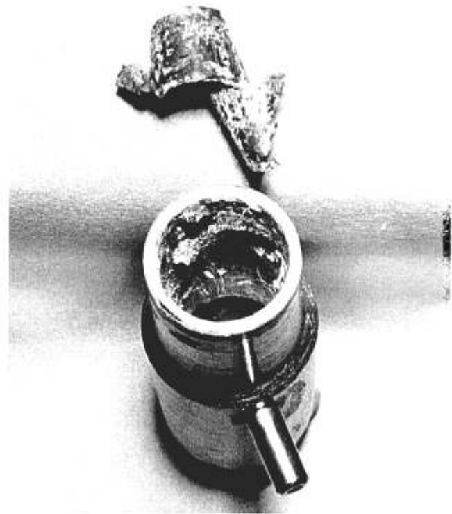
FIG. 1. Corroded T-piece with coil of dislodged metal plating.
