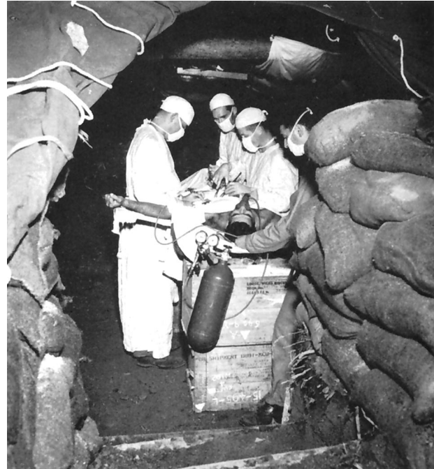
Fig. 6. Underground surgery. The floor is 4 feet below the ground level, the sides are built up with sandbags, and the space is roofed with heavy logs. 21
