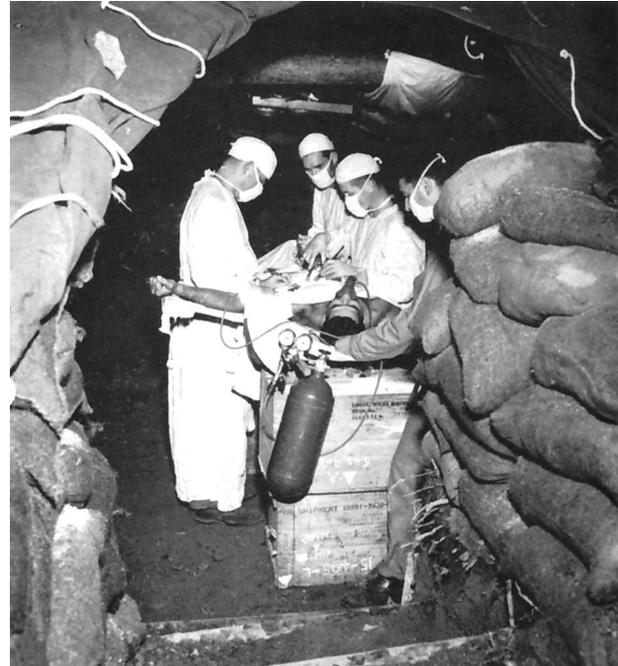
**Fig. 6.** Underground surgery. The floor is 4 feet below the ground level, the sides are built up with sandbags, and the space is roofed with heavy logs.<sup>21</sup>
