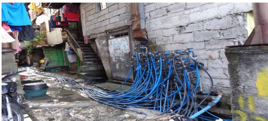
Fig. 4. Typical community-based water reticulation system. *Source*: Photograph taken by author.
