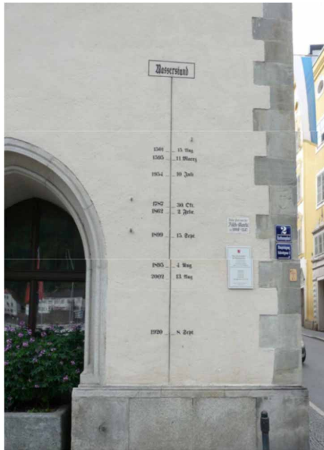
Fig. 2 | High-water scale (1501–2002) taken in 2012 at the tower of the Altes Rathaus, Passau, Germany, as of September 2012 (Eychaner, 2015). Reproduced with permission of the Association of State Flood Plain Managers.
