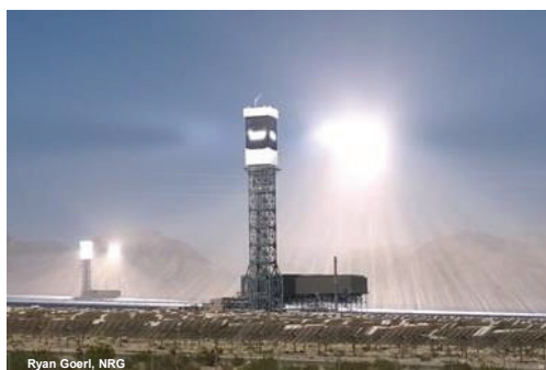
FIGURE 3. Illuminated standby aim points near the receiver at ISEGS before changes were made to spread the standby aim points to reduce the concentrated flux.
