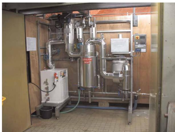
Figure 1 | Pilot thermal sludge hydrolysis (Cambi) at Hengelo WWTP.
