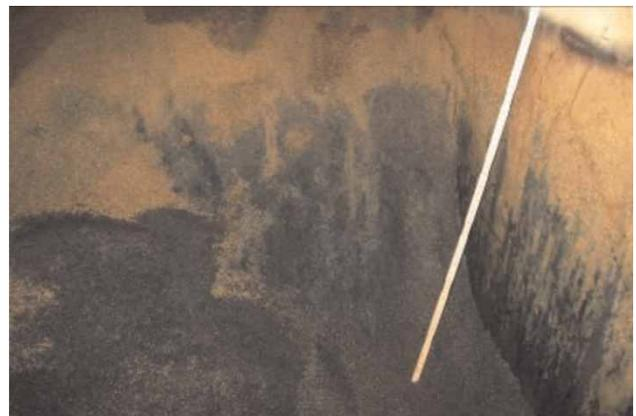
**Figure 2** | Picture of filter media from a second stage rapid sand filter at a Danish groundwater treatment plant. Layers of sand of different colors and grain sizes are mixed, without the expected horizontal stratification.
