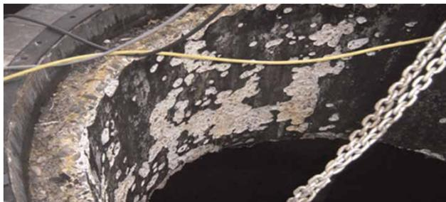
Figure 1 | Concrete corrosion pattern observed in the headspace of digester E.
