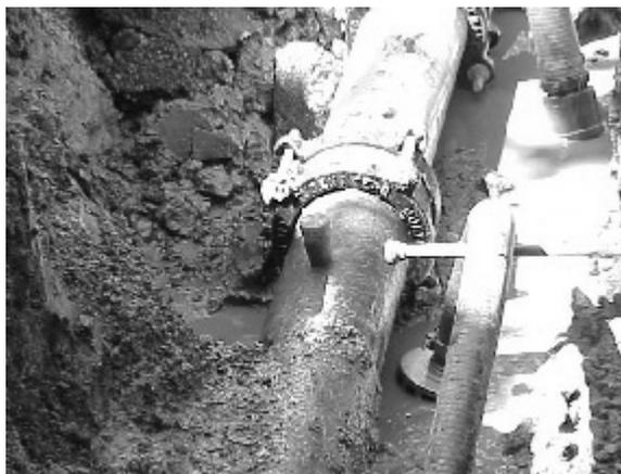
**Figure 2** The typical process of using a peg to repair a perforated water main.
