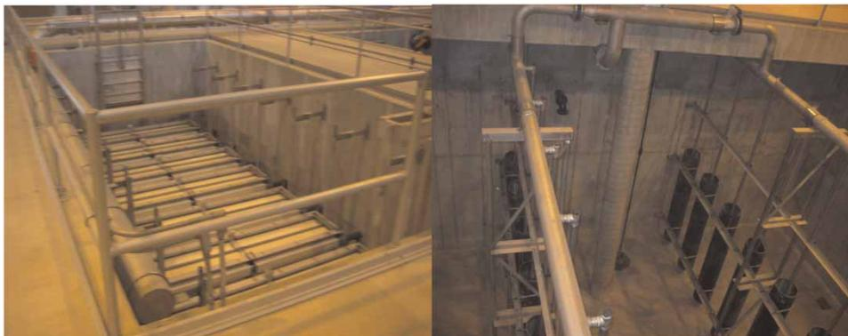
**Figure 5** | Union Rome WWTP membrane thickening aerobic digestion system (MBT shown on the left, aerobic digester shown on the right).
