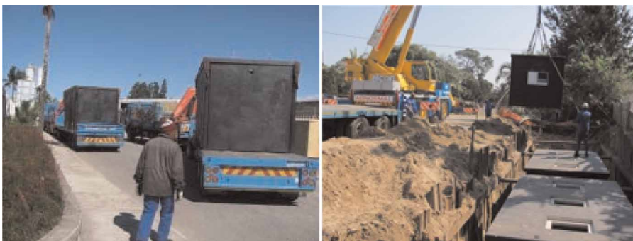
Figure 4 | Transportation and installation of prefabricated packages in South Africa.
