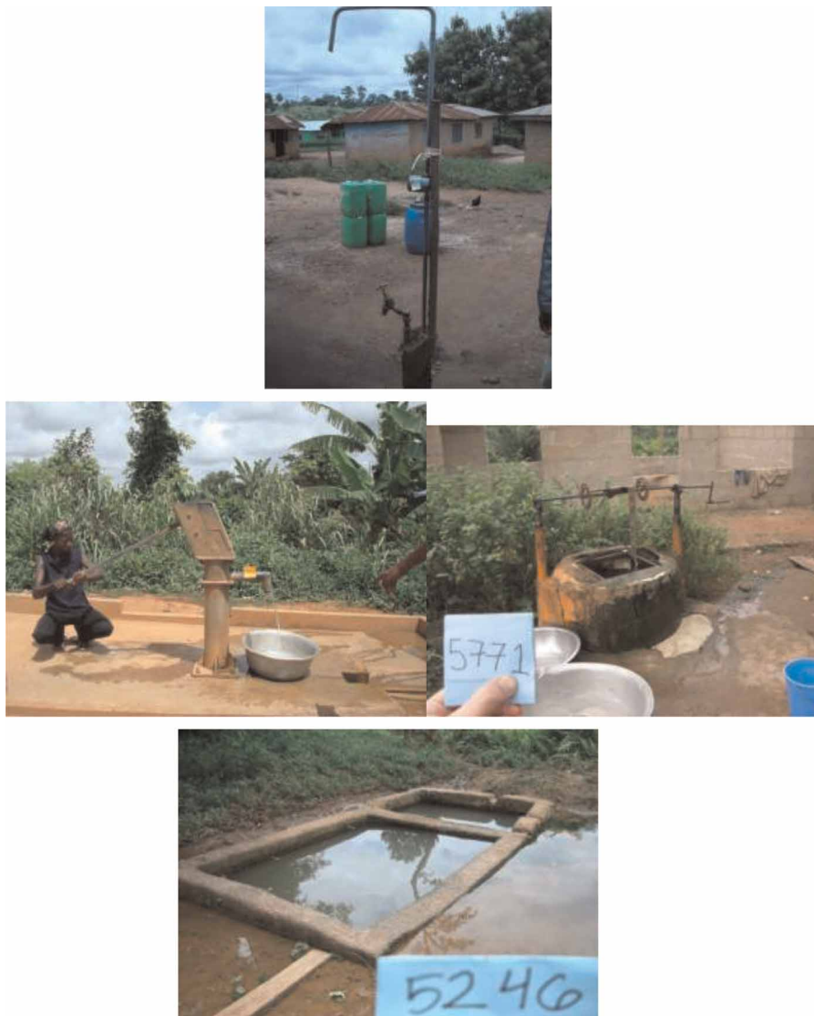
Figure 1 | Examples (clockwise from top left) of a standpipe, borehole, shallow well, and a dug well in the Barekese sub-district, Ghana.
