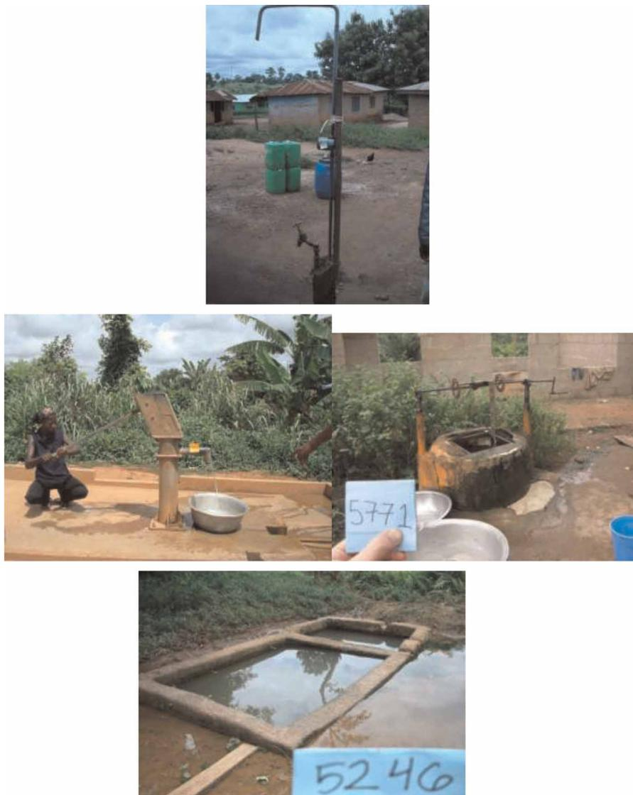
**Figure 1** | Examples (clockwise from top left) of a standpipe, borehole, shallow well, and a dug well in the Barekese sub-district, Ghana.
