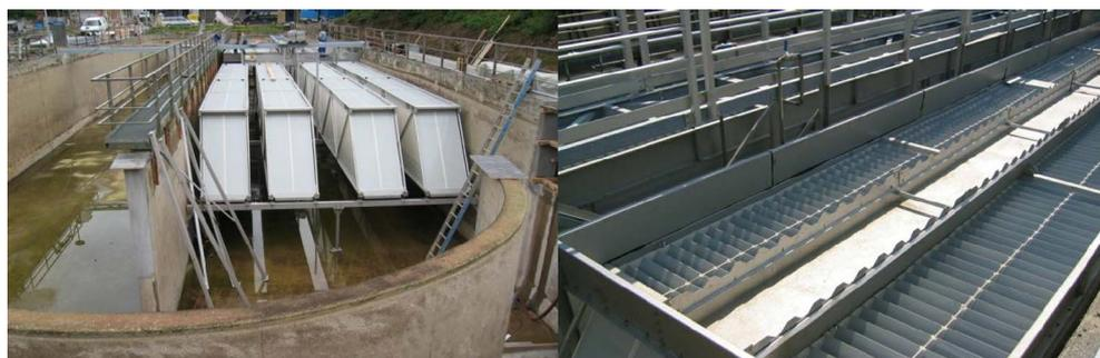
**Figure 4** | Installation of lamella separators in the activated sludge tank.
