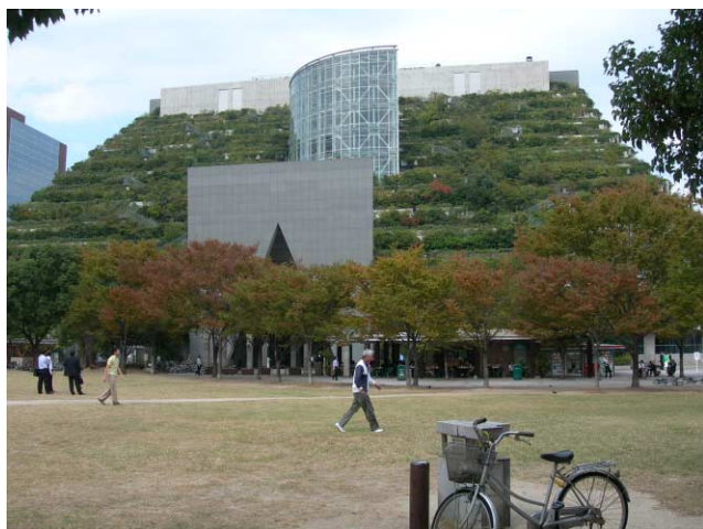
Figure 2 | Vegetated terraces at ACROS building (roof J), Fukuoka, Japan.
