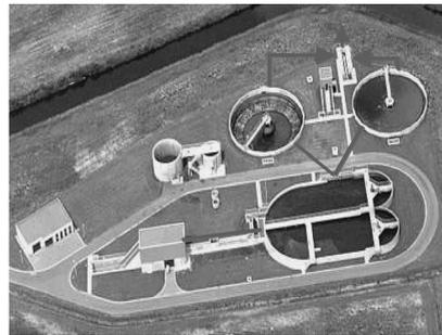
**Figure 1** STP Ertvelde – conventional operation with stormwater tank (left) versus high-flow operation with extra clarifier (right): 1 clarifier + 1 storm tank => 2 clarifiers
