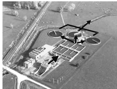
**Figure 2** STP Tielt – conventional operation with stormwater tank (left) versus high-flow operation with extra clarifier (right): 2 clarifiers + 1 storm tank => 3 clarifiers
