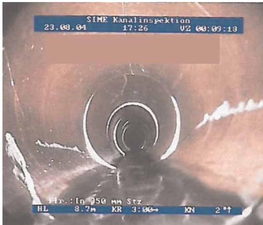
**Figure 3** | CS 4. Damage in stoneware sewer pipe, circular shaped; construction year 1906.
