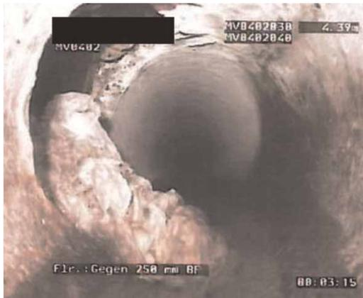
**Figure 2** | CS 3. Damage in concrete sewer pipe, circular shaped; construction year 1906.
