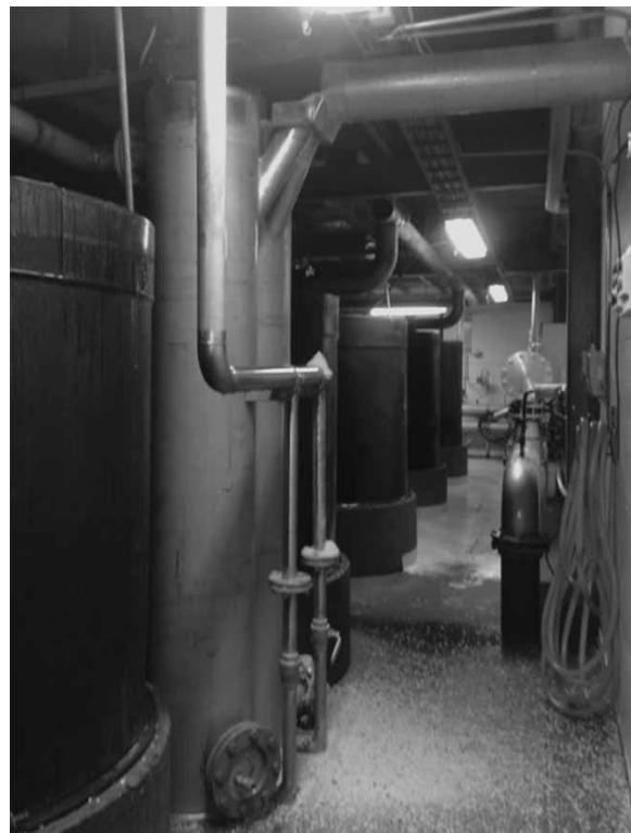
**Figure 3** | Limestone grinders in the Haukipudas groundwater treatment plant. The black tanks each contain 28 rock wool cartridge filters.
