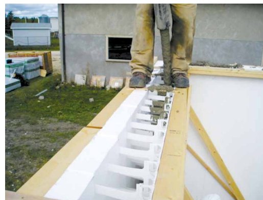
FIGURE 4. Pumping concrete into PVC stay in place Wall System.
