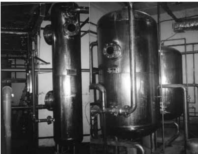
**Figure 2** | Ozone contact column (left), BAC filter (middle) and Muyushi/sand filter (right).
