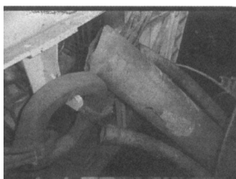
CLOSE UP OF RISER JOINT NO. 1
