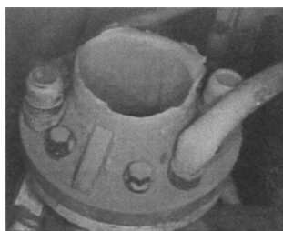
TOP OF LOWER MARINE RISER PACKAGE (LMRP) WHERE JOINT NO. 1 HAD BEEN CONNECTED
