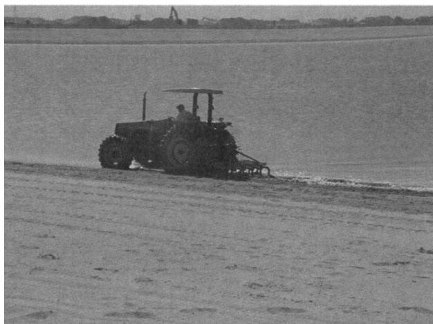
FIGURE 6. TYPE OF RAKING PERFORMED ON LIGHTLY OIL-CONTAMINATED AREAS.
