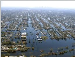
Hurricane Katrina, 2005. Photo courtesy of USCG.
