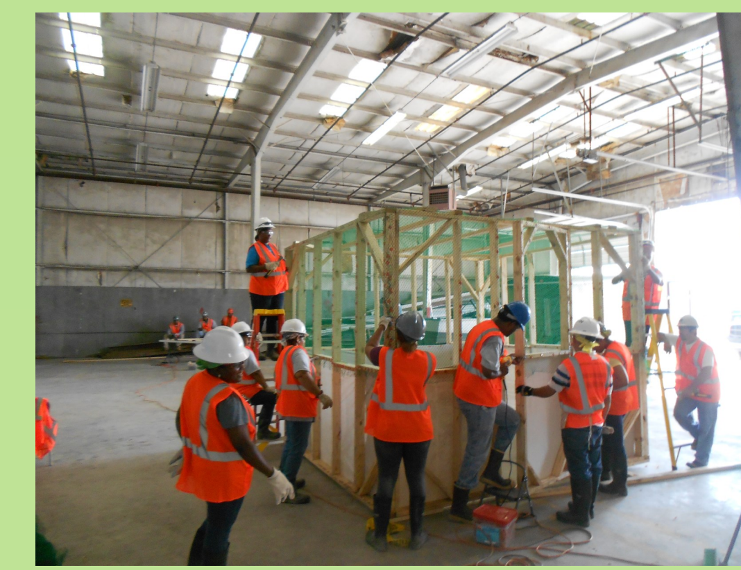
Construction of Wildlife Holding Pens
