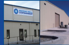
Construction of MCV and SURF Shore Bases completed
