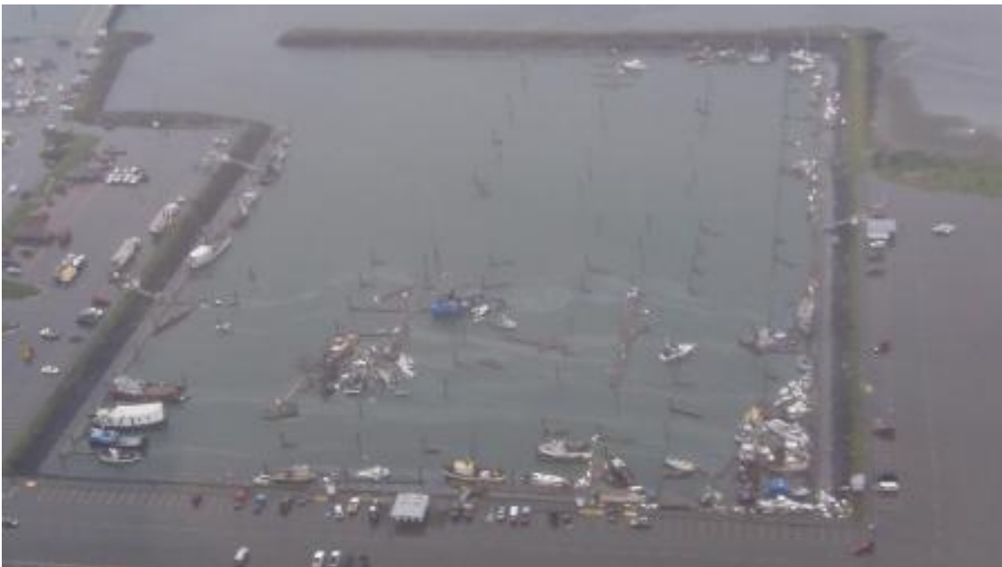
Figure 3 - Crescent City inner boat basin post tsunami surges (USCG)
