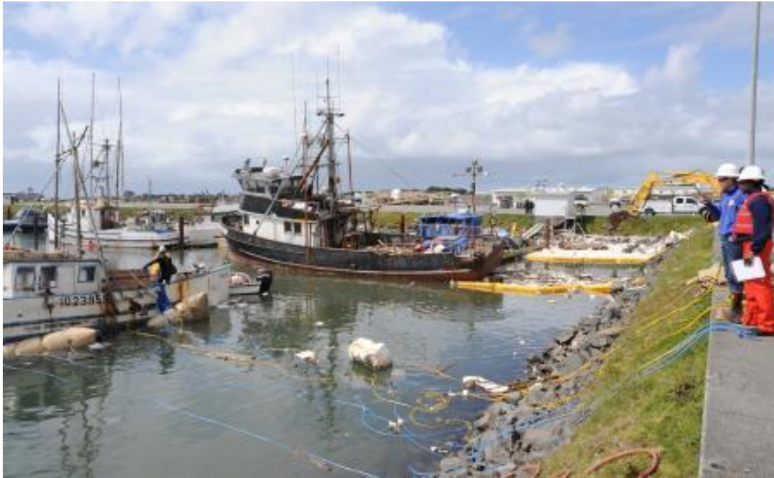
Figure 4 - Assessment of damages in Crescent City (USCG)
