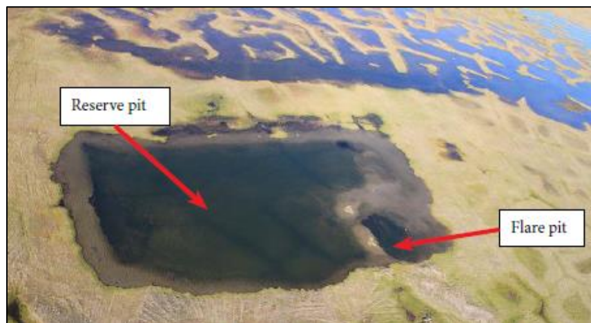
Figure 8: An aerial photo of South Simpson #1, showing the collapsed berm between the flare and reserve pits (US BLM, 2013).
