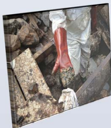
CTO from the spill in Söderhamn is being cleaned-up from inside a jetty
