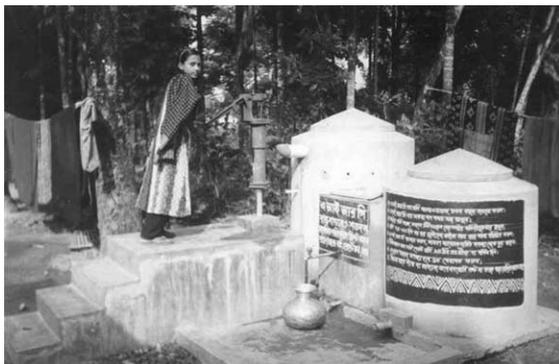
Figure 2 | Typical community arsenic and iron removal plant.
