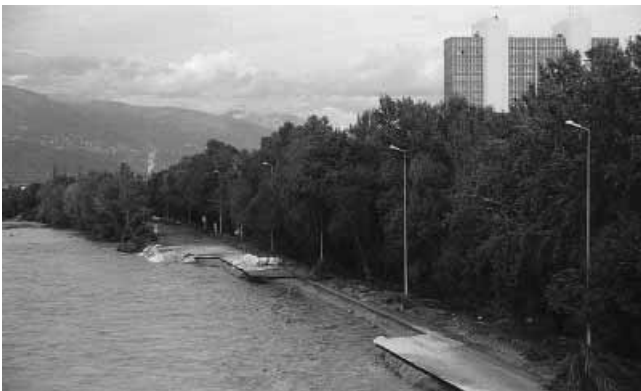
Figure 9 | Downstream area of the Var valley, 6 November 1994 (picture: Nice Matin).
