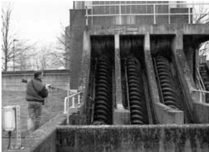
**Figure 3** Illustration of the sound measurements and typical configuration of screw pumps at the WWTP Hove (to be renovated)
