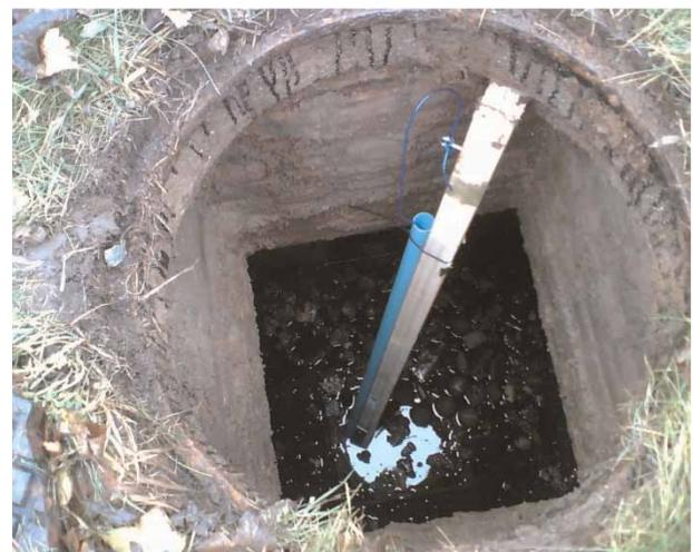
**Figure 3** | Picture of an installed sensor in a manhole. The CTD-diver is in a protective tube (note the gross solids in the manhole).
