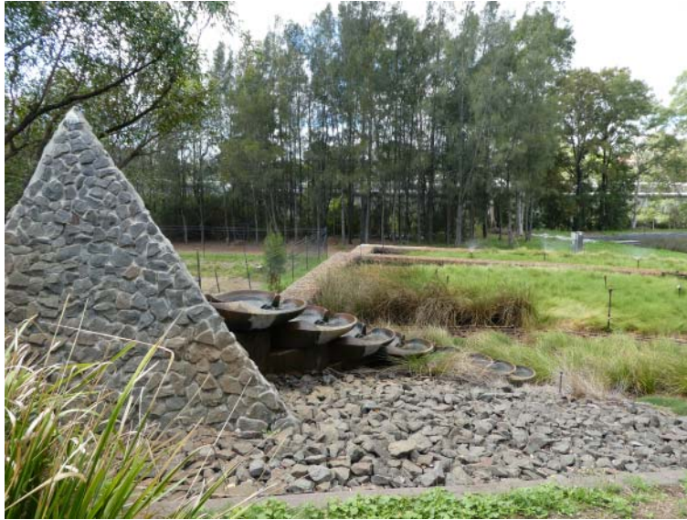
Figures 5 and 6. (Top) Green and golden bell frogs spontaneously emerged in polluted water at the Blaxland Landfill Leachate Treatment facility. (Bottom) Water from nearby landfills is treated here in a series of bioremediation pools. Silverwater Correctional Complex is visible in the background, behind a row of trees and a razor wire fence. Blaxland Riverside Park, on the opposite side of the prison, has a skate park and a playground on top of a remediated landfill. Photographs by Elizabeth Lara and James Nguyen; published with permission from the Sydney Olympic Park Authority.
