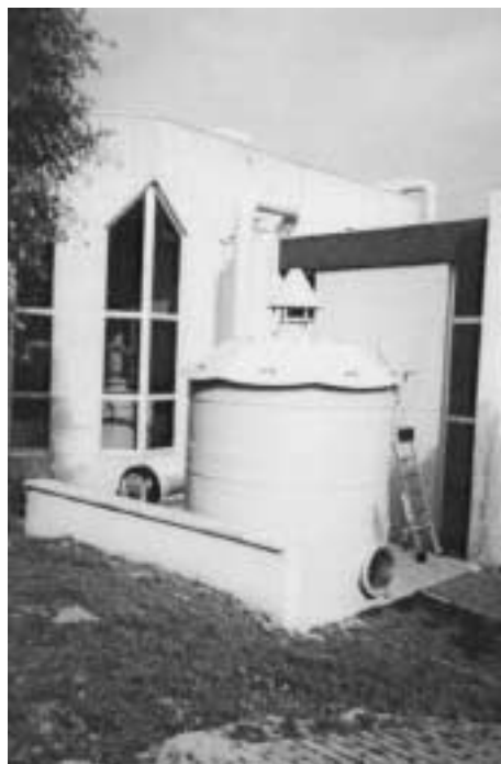
Figure 2 Alizair trickling filter at Le Touquet's WWTP in the north of France
