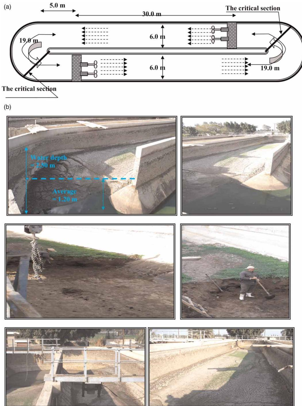
**Figure 1** | (a) OD with the critical section. (b) Typical sludge accumulation pattern inside the OD.
