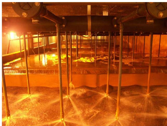
**Figure 2** | Oasen DW trickling filters in production (in the front) and during backwash (in the background).
