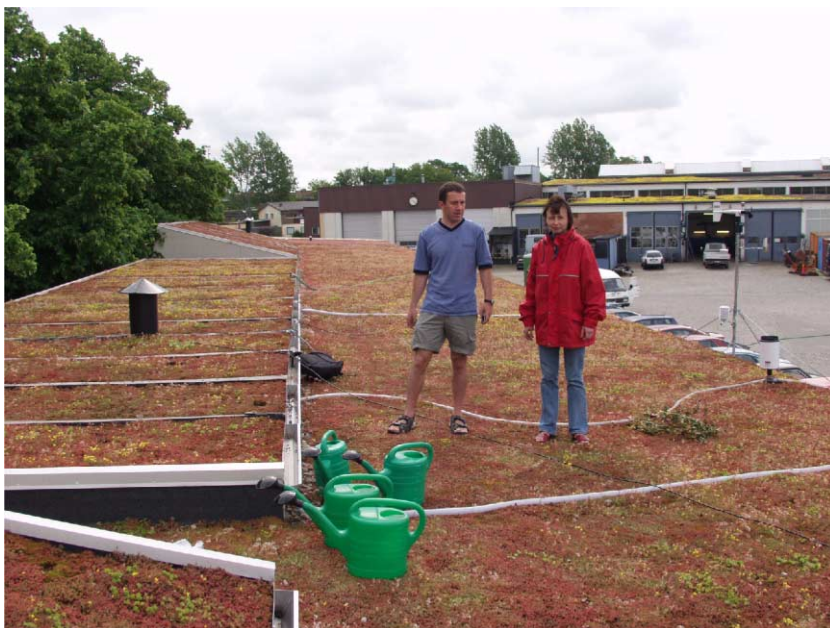
Figure 1 Photo of the experimental roofs at Augustenborg. The hoses lead to barrels beneath the roof. The meteorological station is to the right
