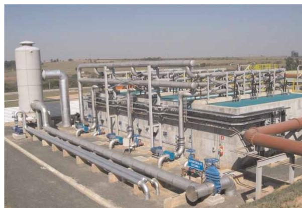
**Figure 4** | View of the three membrane trains and ancillary equipment at the SANASA EPAR Capivari II MBR plant.
