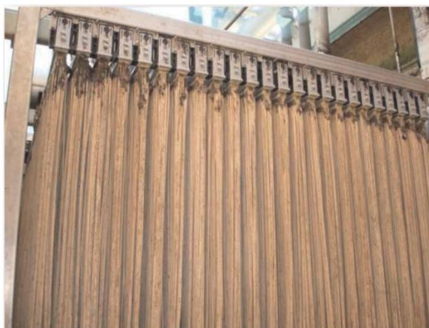
**Figure 5** | Membrane fibers after 1 year of uninterrupted operation: absence of broken fibers and sludge/solids accumulation among them.
