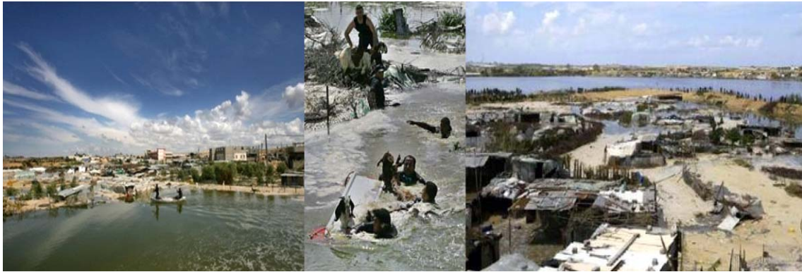
Fig. 2. The flooded Beit Lahia Wastewater Treatment Plant (March 2007).
