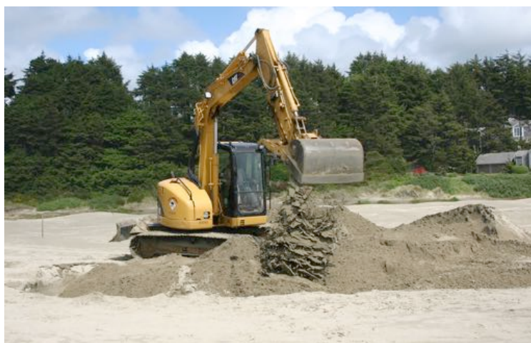
Figure 7. The excavator fills the hole back in with sand. Photo: Oregon Parks and Recreation Department.
