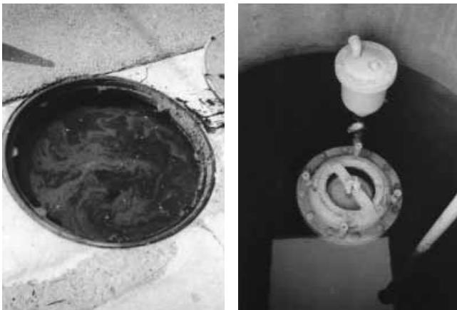
Figure 2 | Submerged air release valve.
