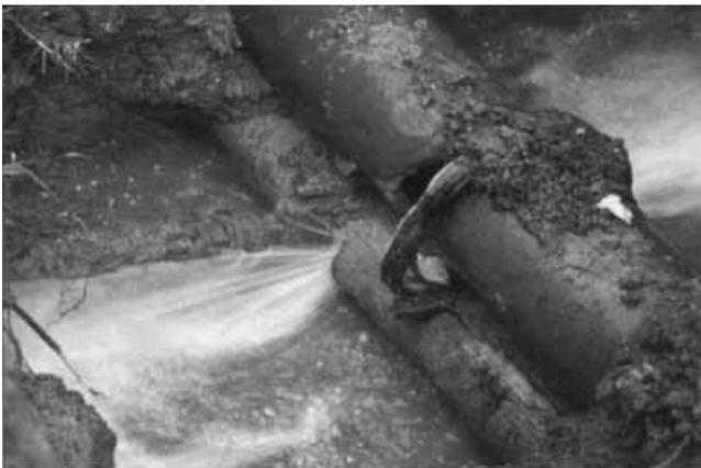
**Figure 4** | Leaky water pipe laid next to a sewer pipe (source: Gary Feeny, Earth Tech. Reprinted from *Opflow* 25(9), September 1999 by permission. Copyright © 1999, American Water Works Association).
