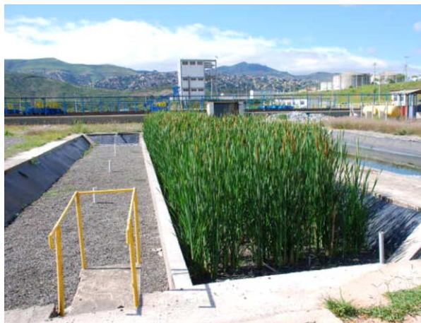
Figure 1 | View of the unplanted and planted subsurface-flow wetland units.
