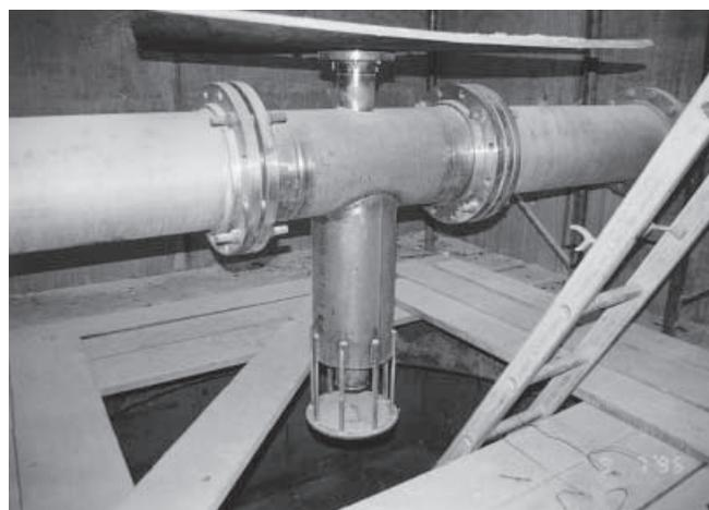
Figure 6 | The flash mixing system during construction.
