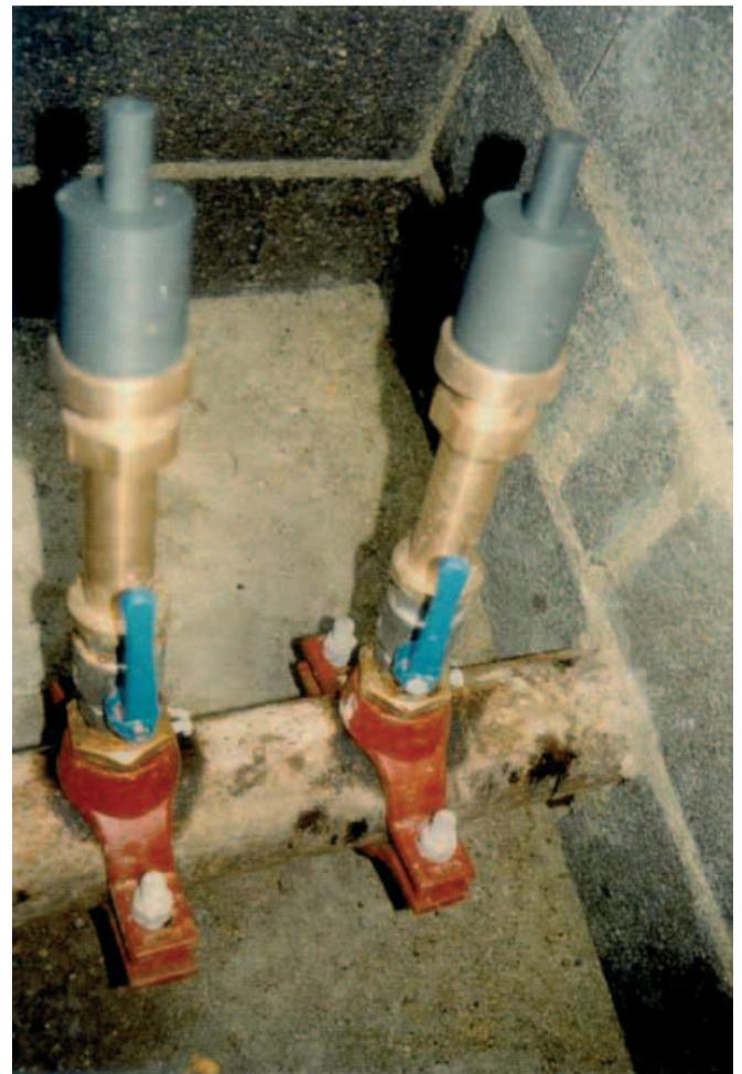
**Figure 2** | View of a chamber allowing direct access to a 100 mm diameter pipe with two sampling devices which permitted the insertion of a cast-iron coupon just at the inner surface of the pipe.
