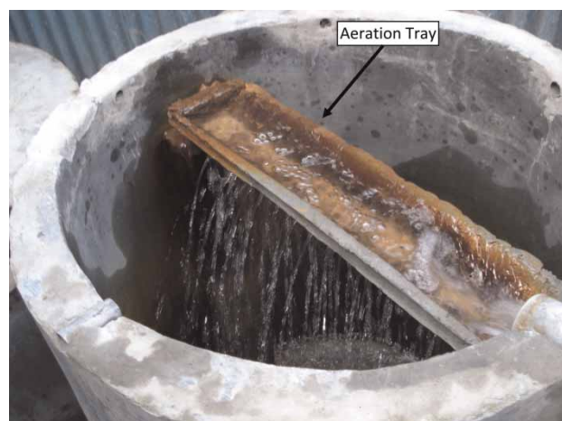
Figure 2 | Inside aeration tank.
