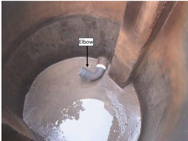
**Figure 5** | Aeration tank with elbow installed.
