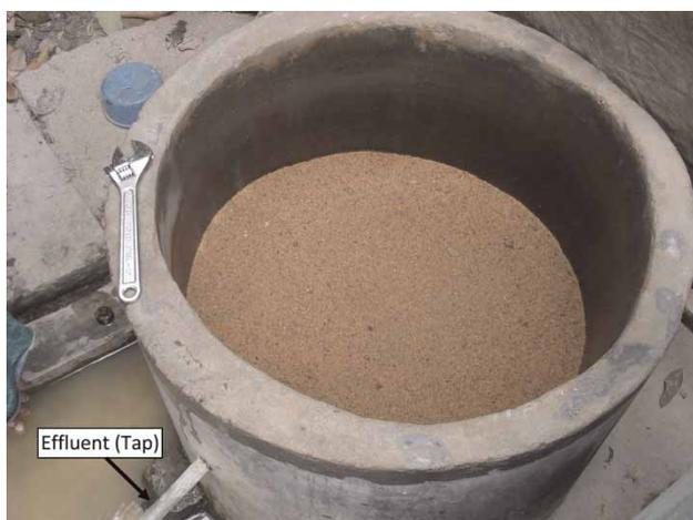
Figure 3 | Filtration tank.
